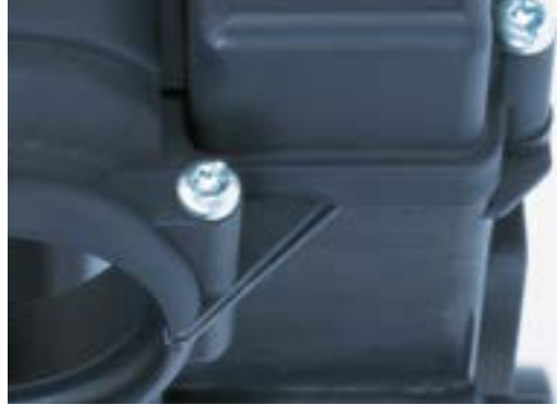
Figure 8.11 Direct screwing into thermoplastic material
